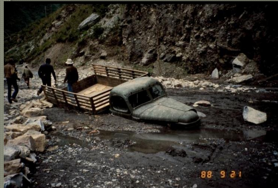
Washed out road
