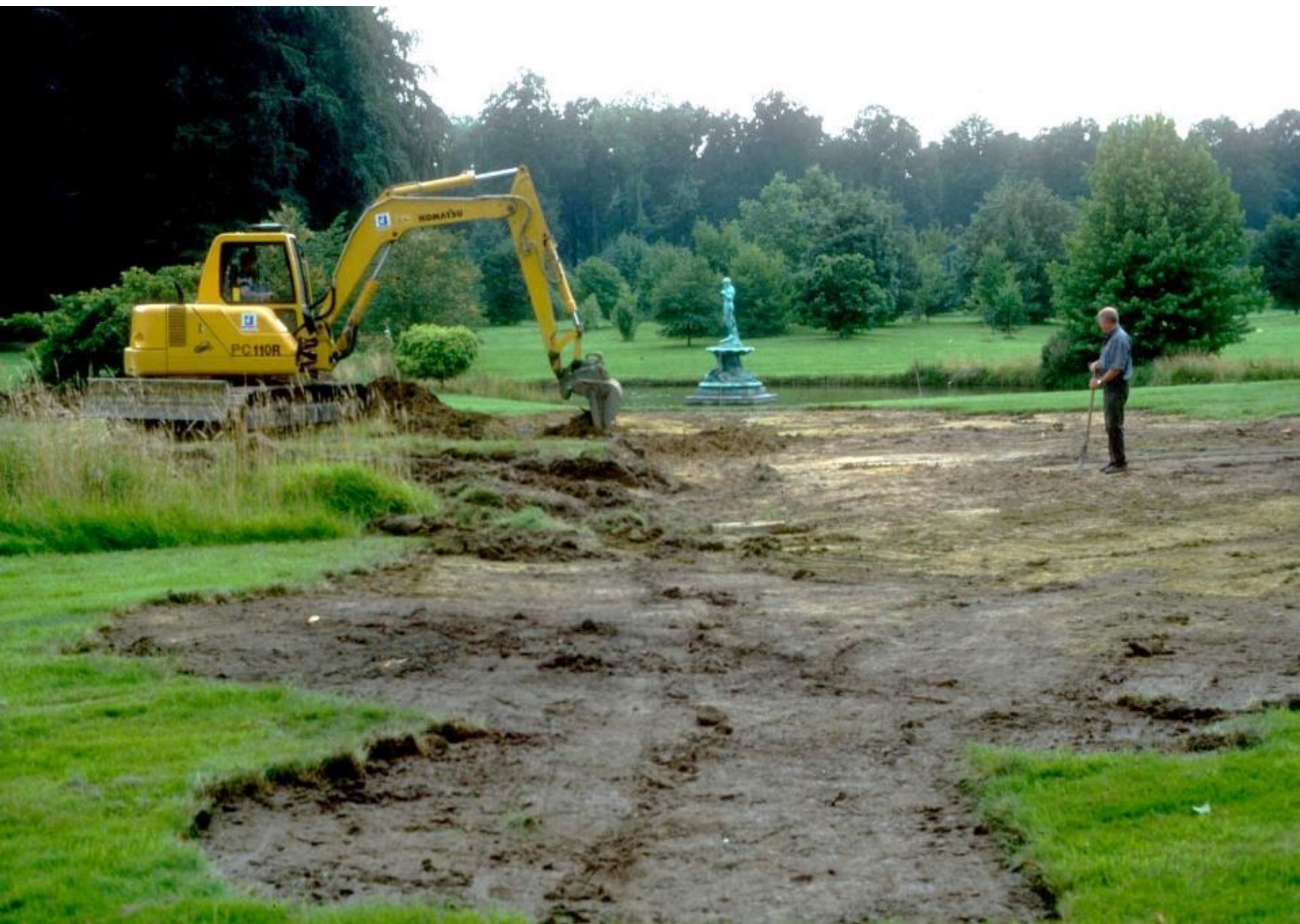
Providing for natural slope draining towards ponds or ditches, and some landscaping effect
